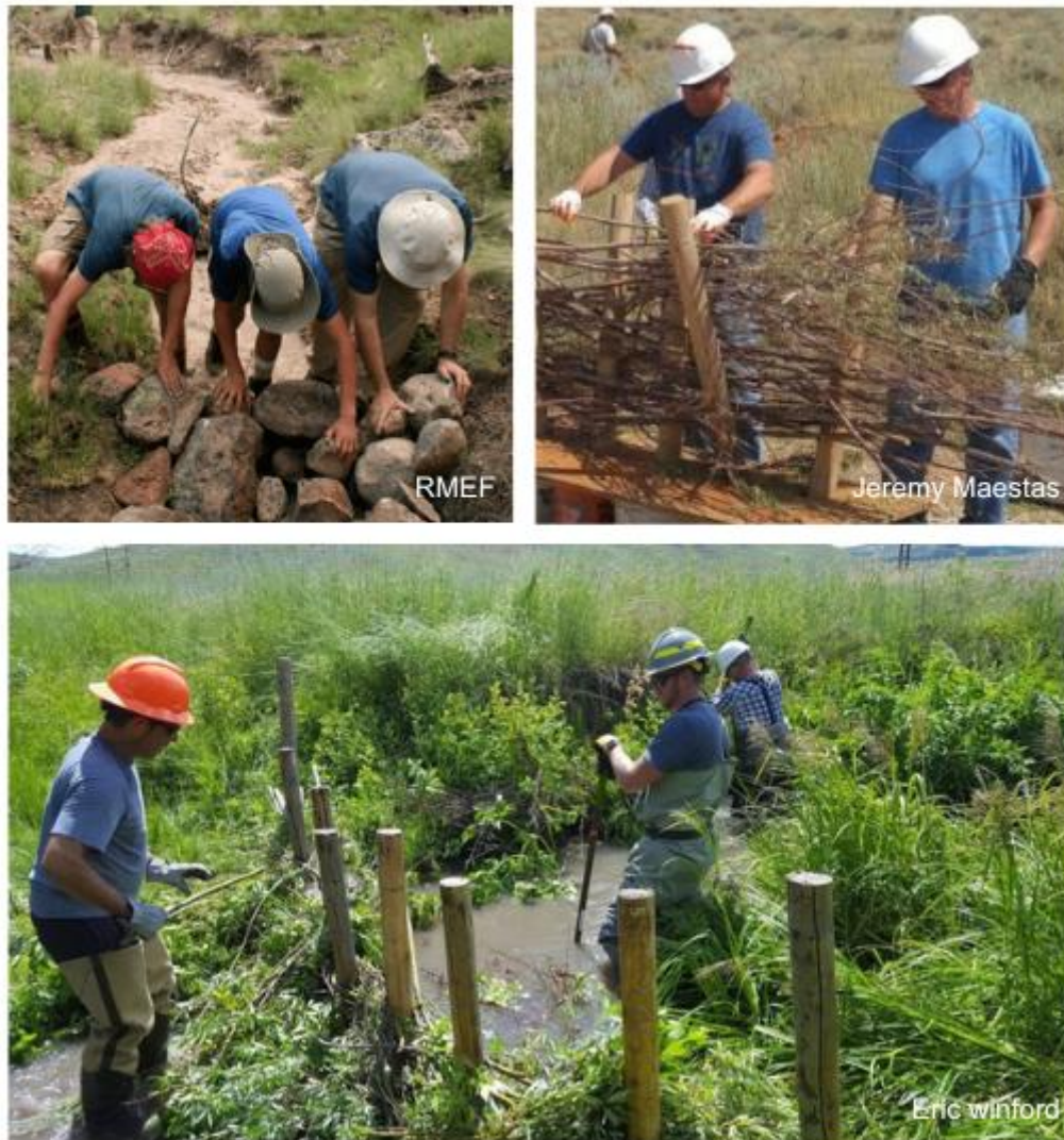
Figure 4: Examples of low-tech, process-based restoration techniques. Images show (bottom) installation of a post-assisted structure or beaver dam analogue (BDA), (top right) weaving of a demonstration BDA, and (top left) construction of a rock Zeedyk-style structure. These structures are installed manually using locally sourced materials, reflecting their low cost, scalability, and ability to mimic natural hydrological processes.
